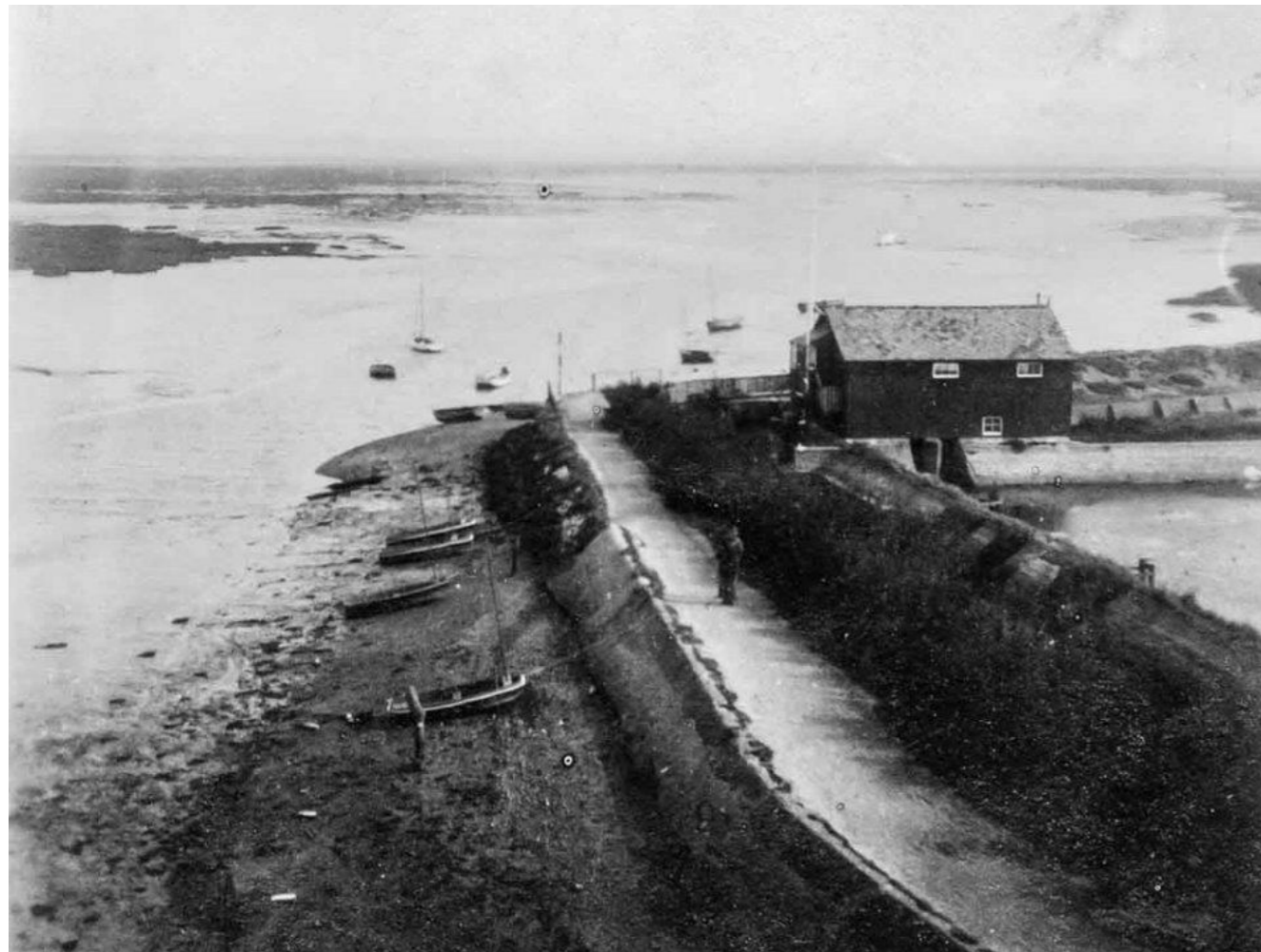
The original site of Hayling Island Sailing Club at Mengeham Rythe. This clubhouse was built in 1929. Image used with kind permission from Belinda Cook.
